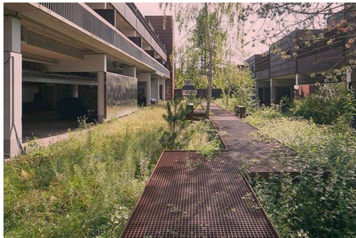
Farum Midtpunkt by Rambøll Architecture and Urban Development
